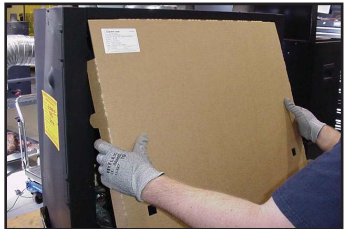
Figure 13.4 Installation of Splatter Guard
